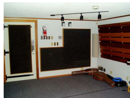
Each room is treated with hand-built Cedar resonators, bass traps, and Sonex.
